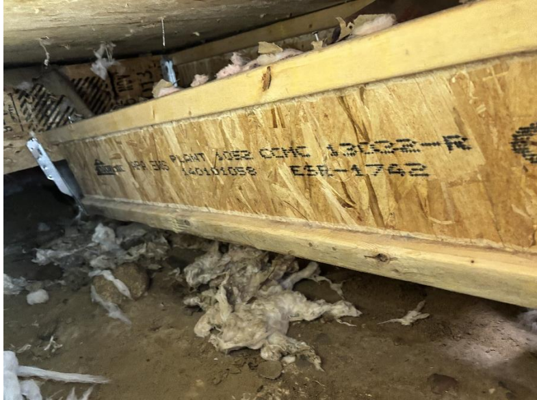
Photo 7: Disconnected I-Joist
