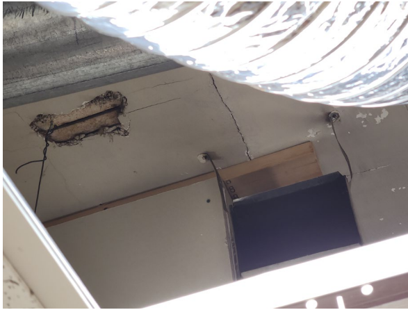
5: The kitchen is VCT 12x12 flooring, possibly c. 1980s plastic laminate. The countertops are chipped, warped, and crooked. The ceiling tiles are not in poor condition however, there is approx. 4-5' above the ACT ceiling, up to the original ceiling, which is lath on plaster. Some of the plaster is missing, and the lath on plaster that remains is terribly cracked. ACT ceiling has 2x4 lights. There is a small hot water tank underneath the microwave next to the window that is roughly 10 gallons.
