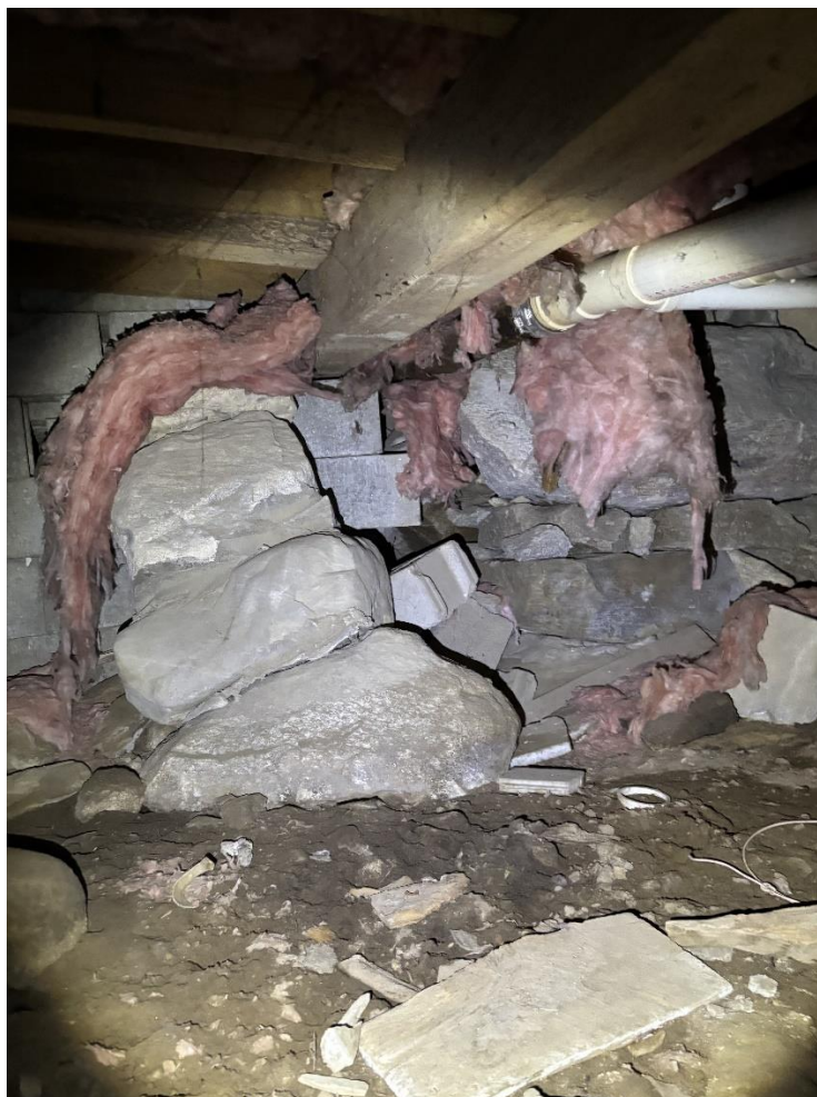
Photo 10: Beam bearing on CMU
