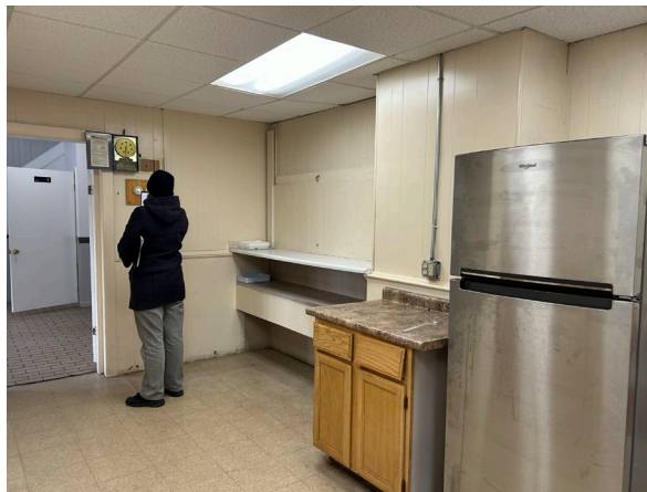
There is a refrigerator, fire extinguisher, surface mounted conduits, two quadruplex receptacle outlets, 70's era wood paneling, which has been painted on the walls. On the wall next to the door is a Dayton seven day dial, time switch, four pole, two normally open, two normally closed, and model number 2E21. The paneling seems original before paint.
