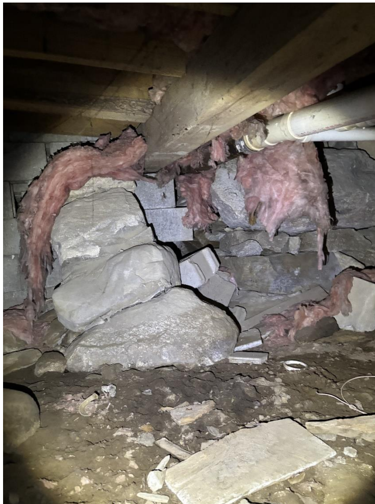
Photo 10: Beam bearing on CMU
