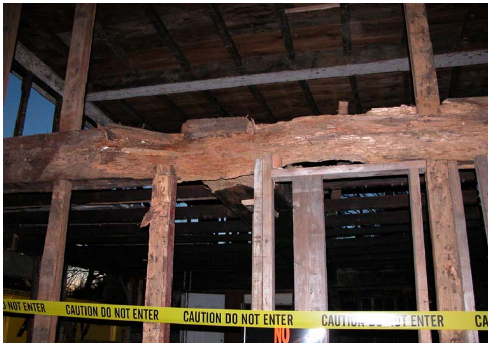
East Gable, Second Floor Girt and Summer Beam
